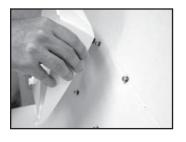
7. Line up the screw heads with the holes on the mounting brackets, and slide the unit down slightly until the screw heads are securely fastened to the mounting bracket.
